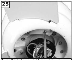
Install blades and blade plates to motor using the 9 motor screws provided. Tighten screws securely.
